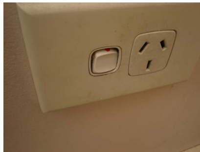
A loose switch to a power point needs repair as soon as possible
