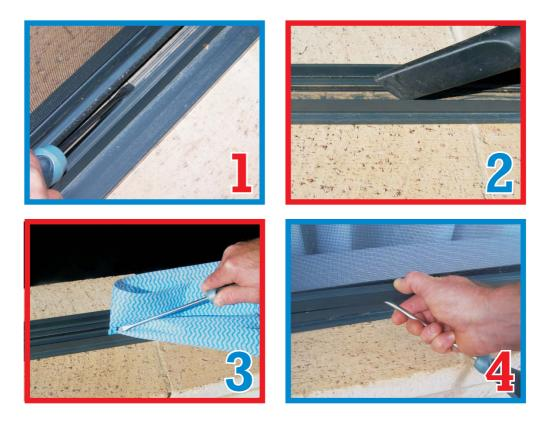
Remove flyscreens by gently placing a screwdriver under the screen, lifting up and sliding to the left or right and pulling out. Do not force screens as they can bend easily. Hose flyscreens if necessary (pic 4).
